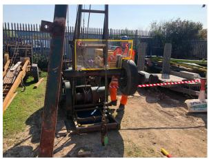
Further engineering controls are provided by establishing two distinct work zones within the standard wider work area. A physical barrier, using either chapter 8 barriers or retractable hi-vis tape attached to magnetic clamps, segregates the work areas of the assistant driller forward of the rig and the lead driller to the rear, and acts to change behavioural patterns by preventing inadvertent close proximity working.
