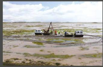
Geotechnics carried out sixteen boreholes over the length of the pipeline route with the Hybrid Hagglund Cable Percussion Rig with boreholes taken to depths
