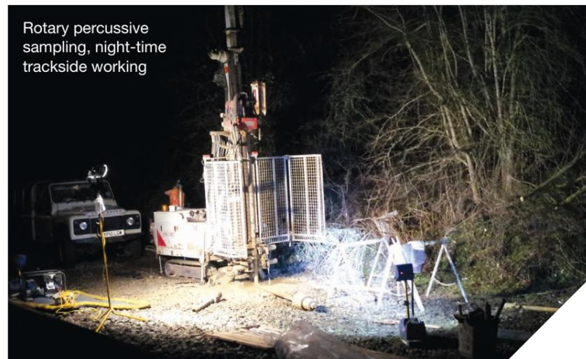
Rotary percussive sampling, night-time trackside working
