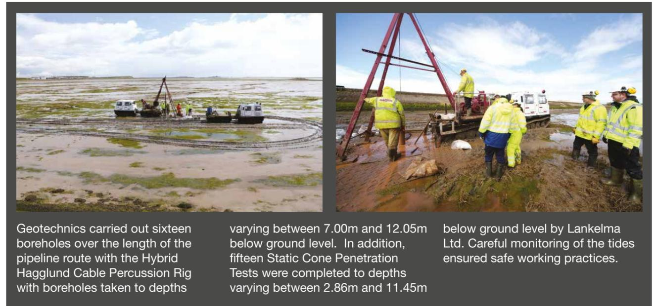
Geotechnics carried out sixteen boreholes over the length of the pipeline route with the Hybrid Hagglund Cable Percussion Rig with boreholes taken to depths
